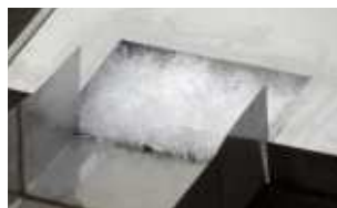
Filtering of waste water before discharging into water discharge area.
