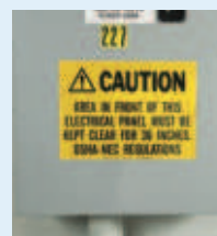
Hazard warning signs
